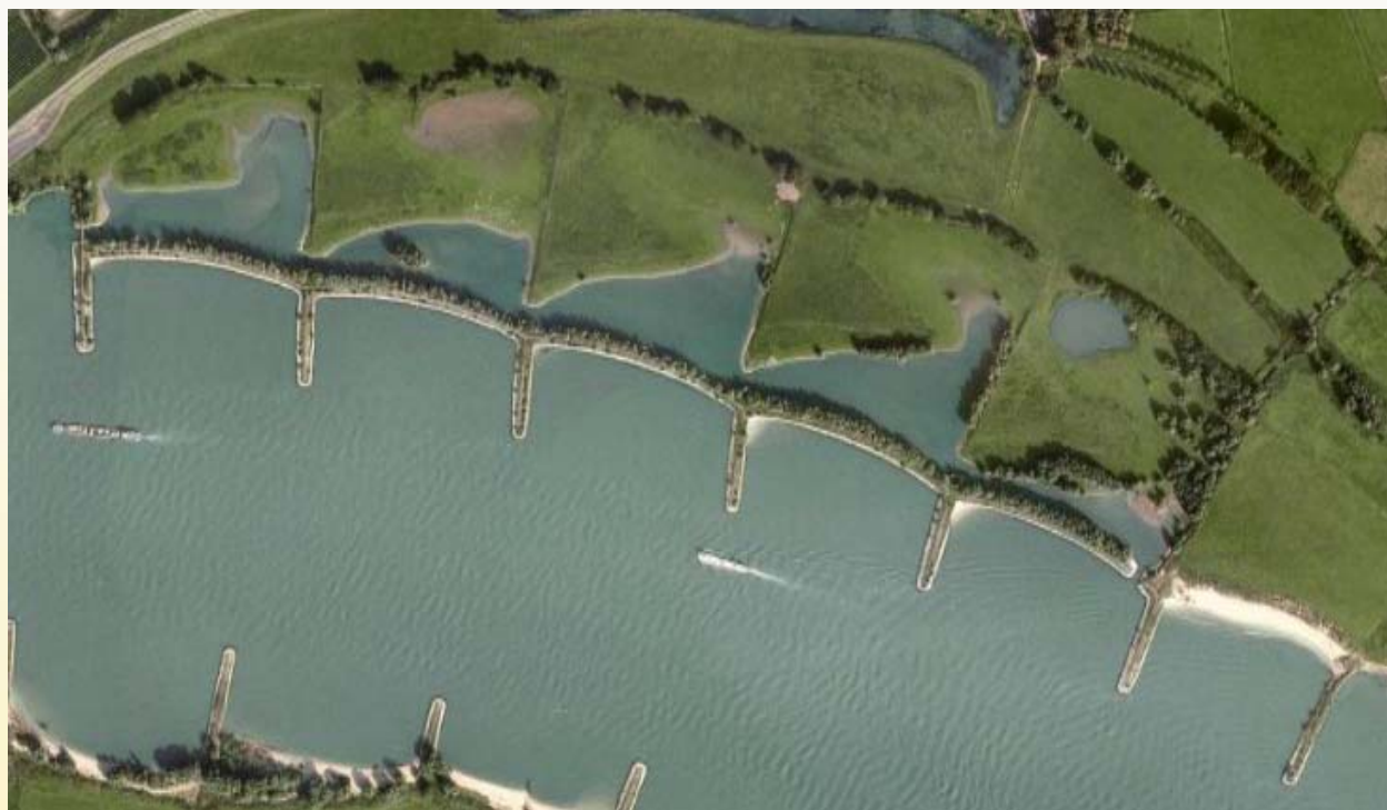
(Groins with off-bank protection Opijnen, The Netherlands)
