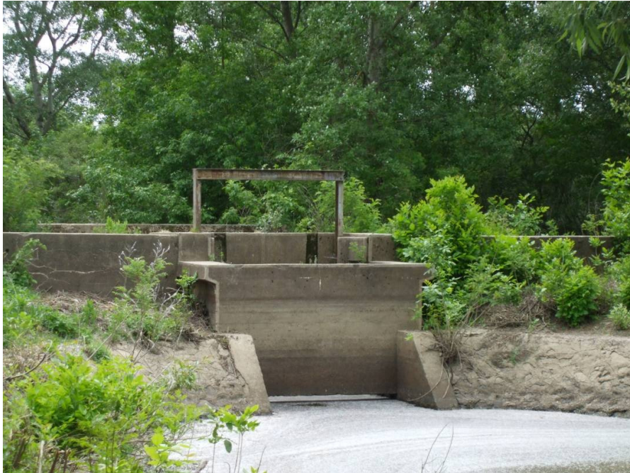
Figure 3: The sluice before renovation
