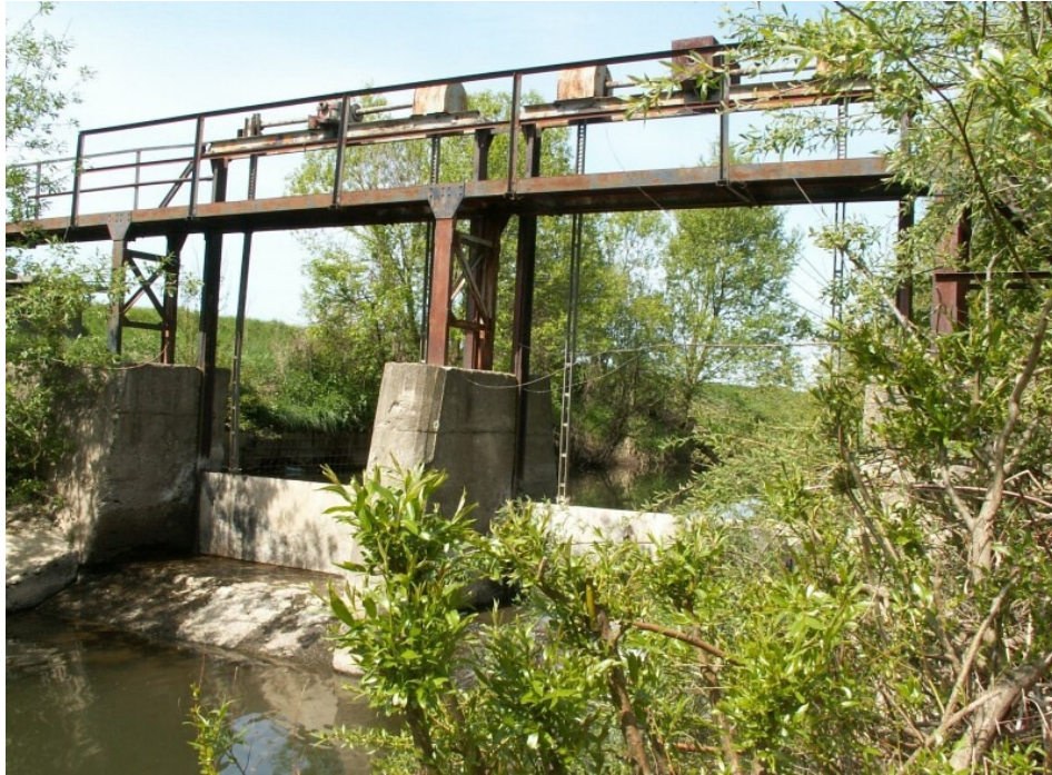
Figure 6: Flood gate before the renovation
