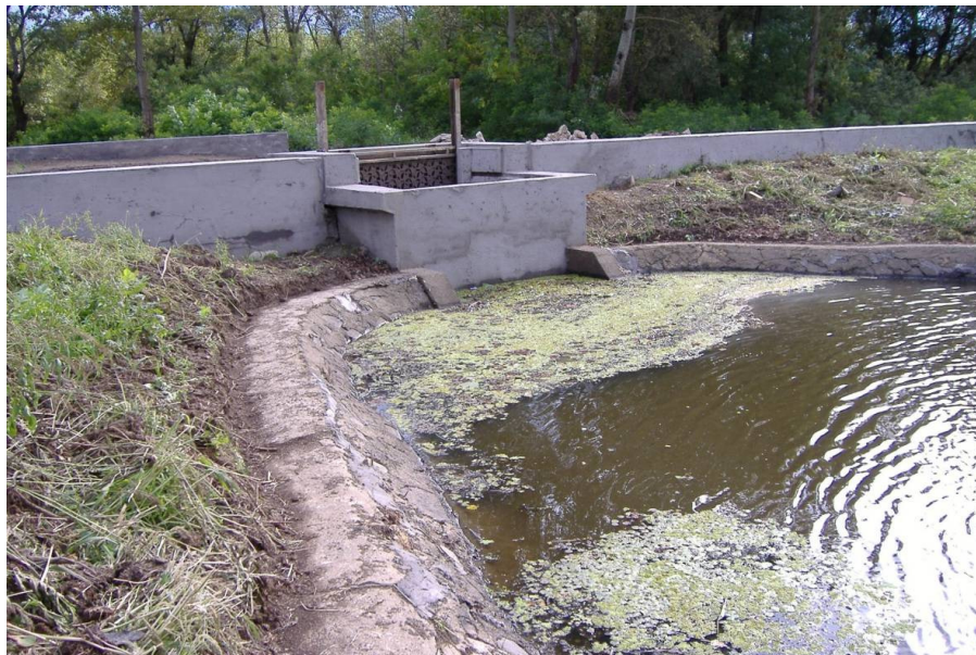
Figure 4: The renovated sluice on Viss Oxbow
