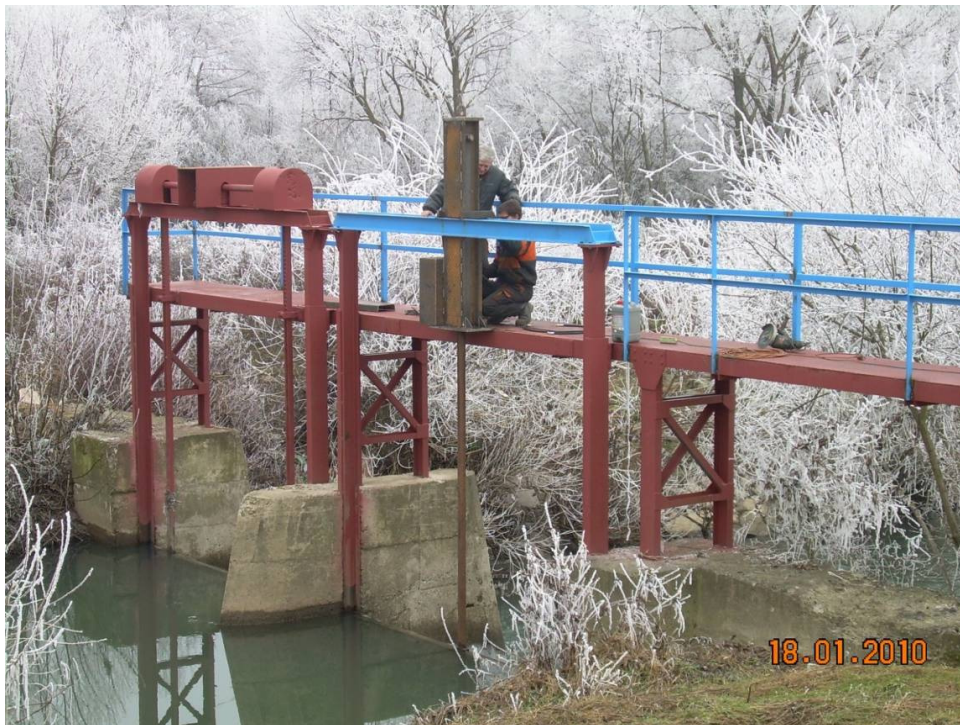
Figure 7: Flood gate after the renovation
