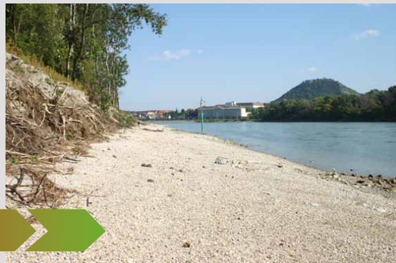
Pilot Project Thurnhausen – renaturated river bank after the construction work. The project was awarded the prize for Best Life Nature Project 2007-2008.
