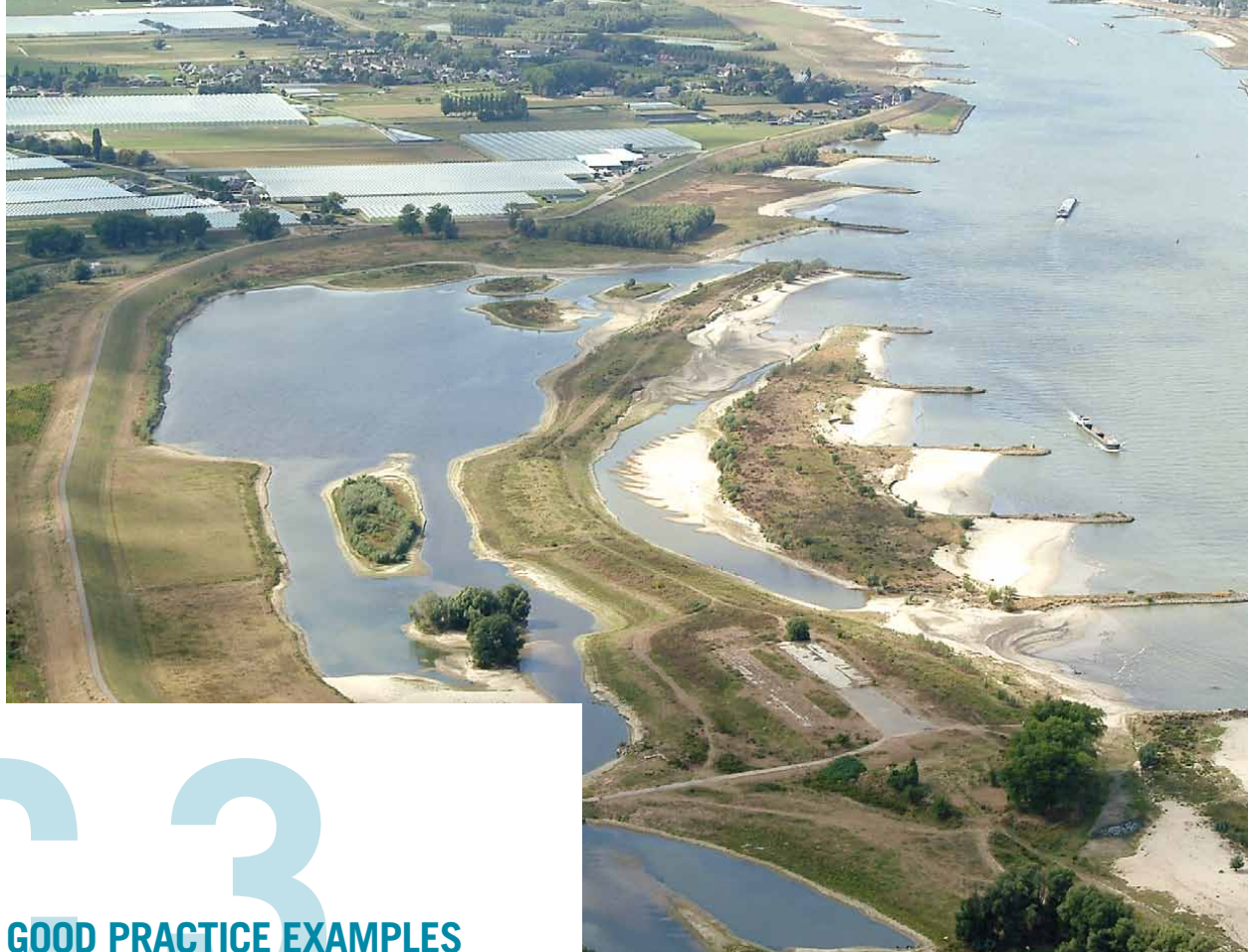
Restoration measures at the Rhine river – Waal branch near Nijmegen (B. Boekhoven (RWS), NL, 2003)
