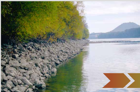
Pilot Project Thurnhausen – bank armoring before construction work.
