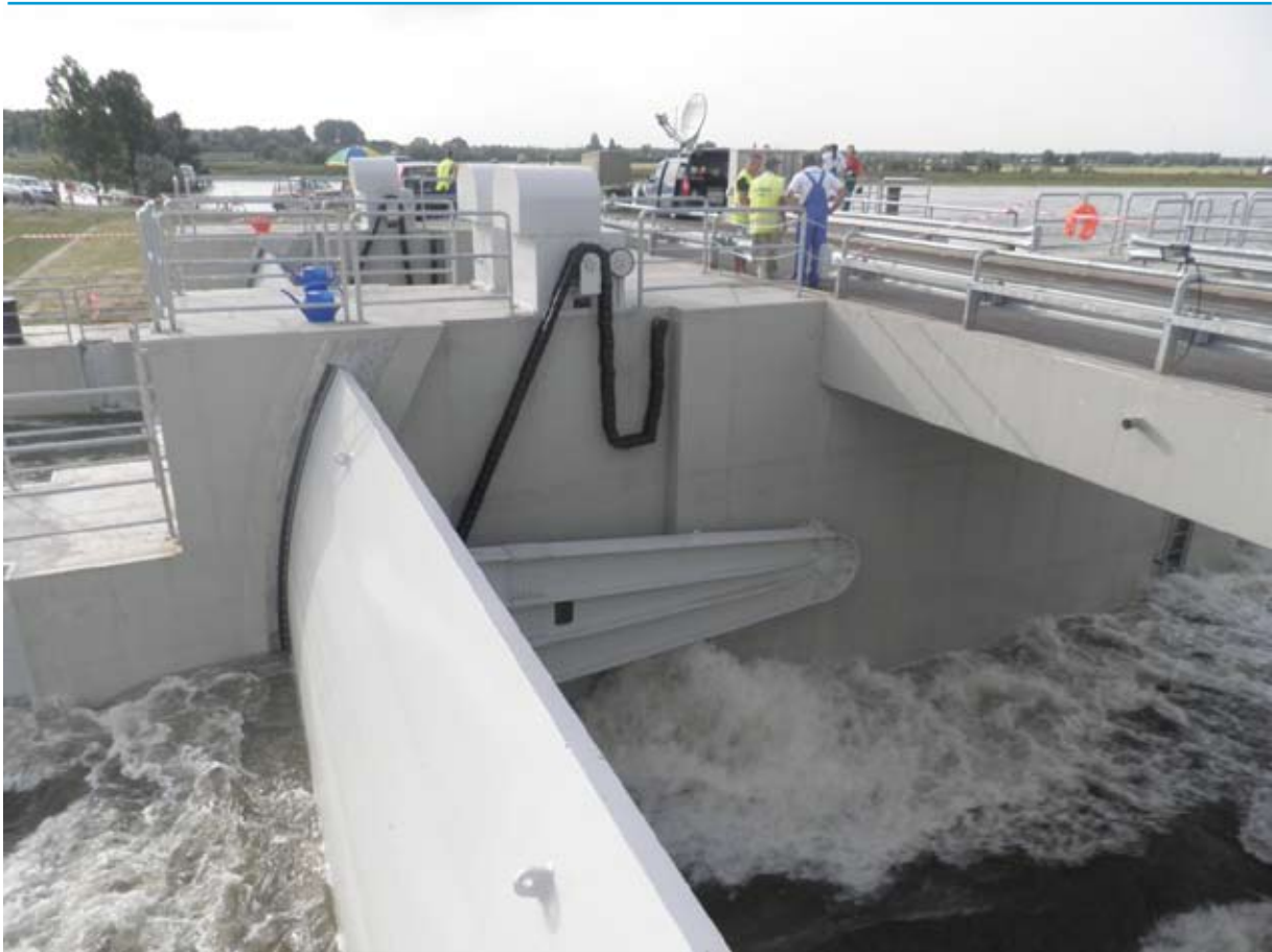
Open locks of the Tiszaroff inlet structure on 14th June, 2010
