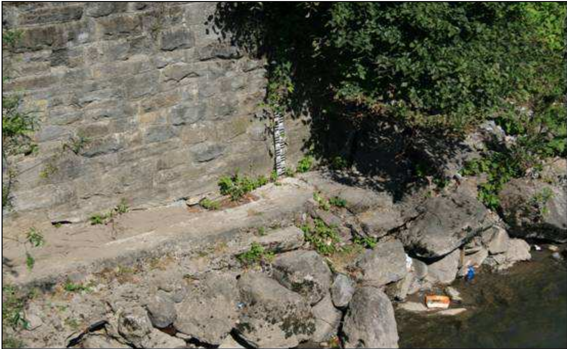
Picture 6. Present state of the water gauging station in Dilove
