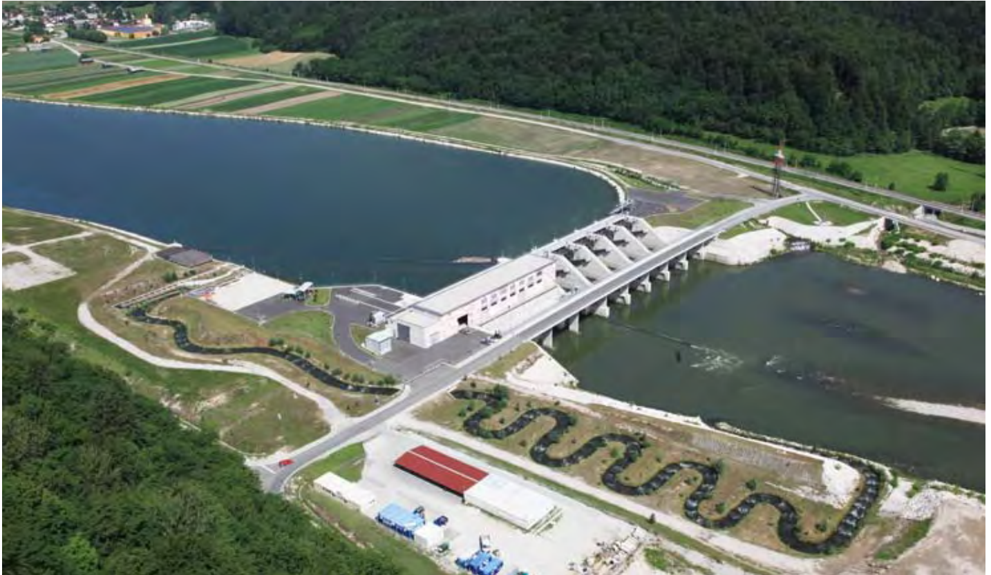
Hydropower plant Arto-Blanca at the Sava River, Slovenia. Hydropower generates renewable energy but also has a negative impact on the environment – the challenge is to strike the right balance. © Hidroelektrarne Na Spodnji Savi
