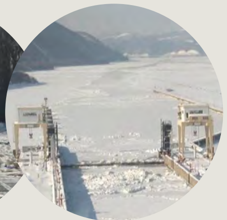
Figure 18: upstream Iron Gates dam, 25 February 2012.
