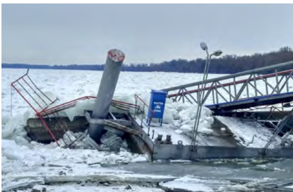
Figure 70: Damaged dock in Apatin
