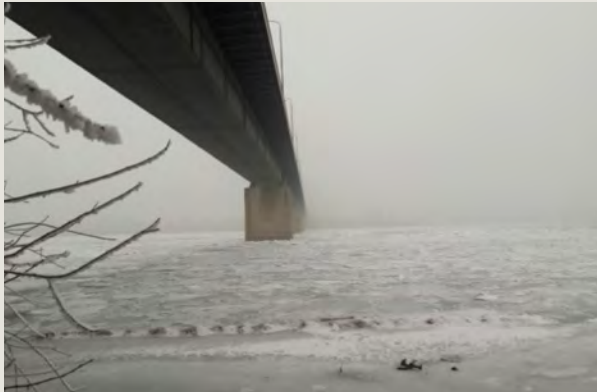
Figure 41: Kovin-Smederevo bridge (km 1112), 25 January 2017
