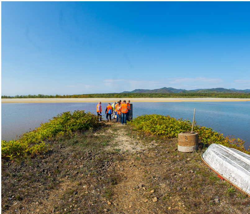
Visual check of the Aurul TMF: decant structure with water level measurement system.
